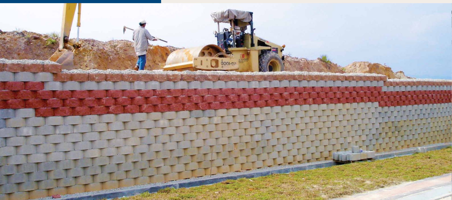
Reinforcing with Miragrid® GX geogrids.
