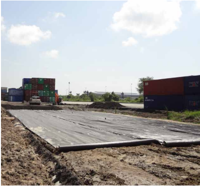
Figure 3: Laying of Mirafi® HPa Geotextile
