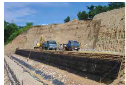
Slope repair works in progress
