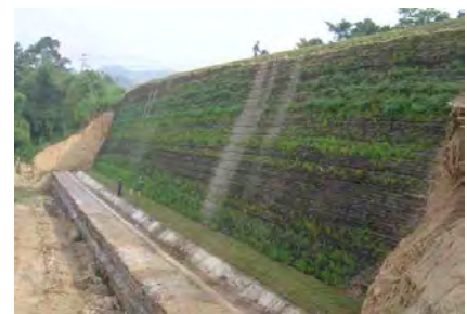
The completed Polyslope B slope with vegetation established
