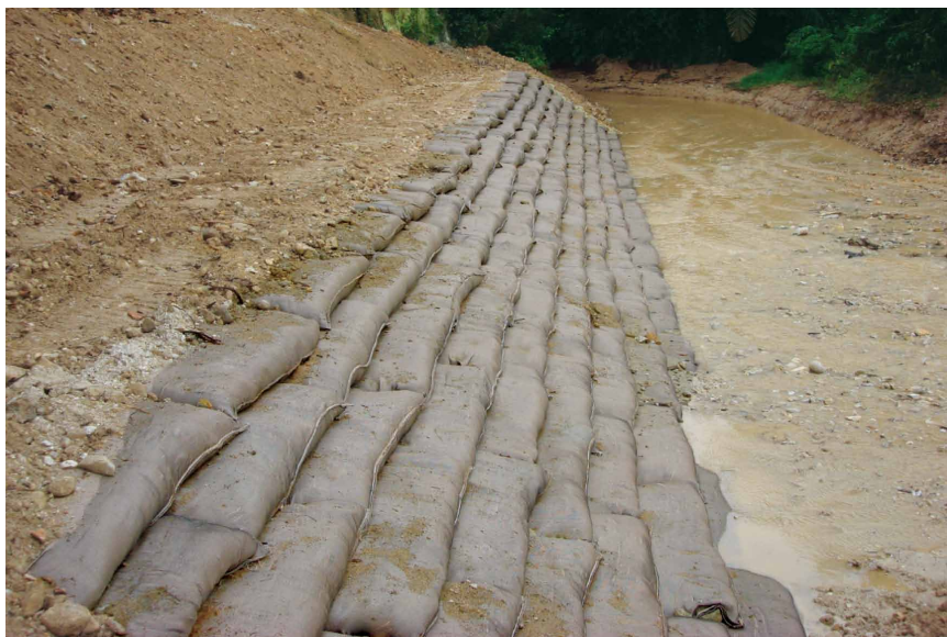
Completed installed geobags at project site.
