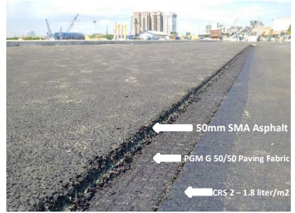
Installed Polyfelt® PGM-G for asphalt reinforcement
