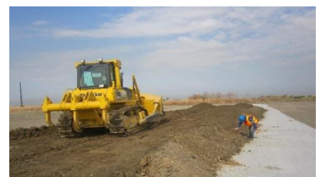
Embankment over Mirafi® PET 100/50 geotextile
