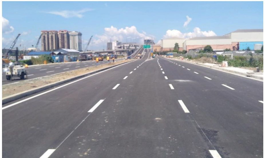
Completed expressway with road base reinforcement
