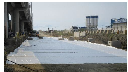
Mirafi® PET 100/50 geotextile laid into soft soil foundation
