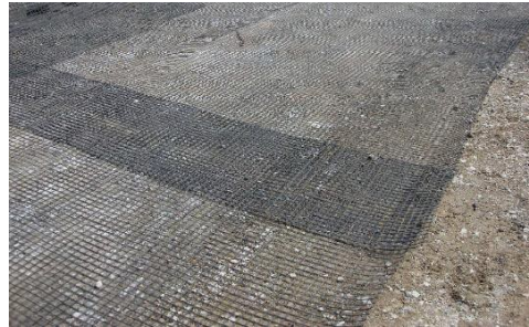
Miragrid® GX geogrids laid after the subbase course
