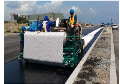
Paving rig used for the lay down of the paving fabric
