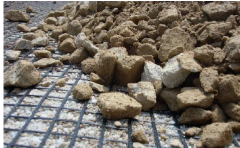
Base course material filled over Miragrid® GX geogrids
