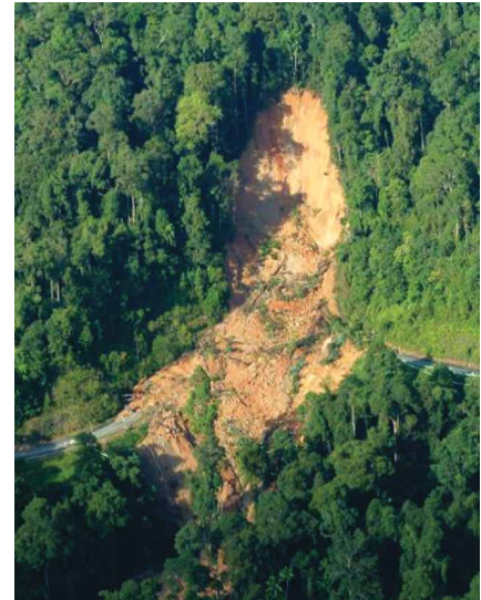
Figure 2: Aerial view of the slope failure.
