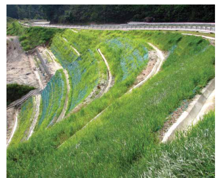
Figure 4: Vegetated slope after completion.
