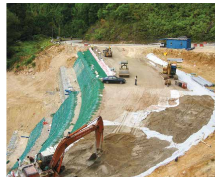
Figure 3: Reinforcing slope with Polyfelt® PEC.
