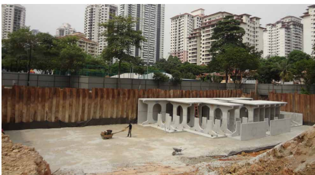
Installation of StormTrap® system over the load transferring platform.
