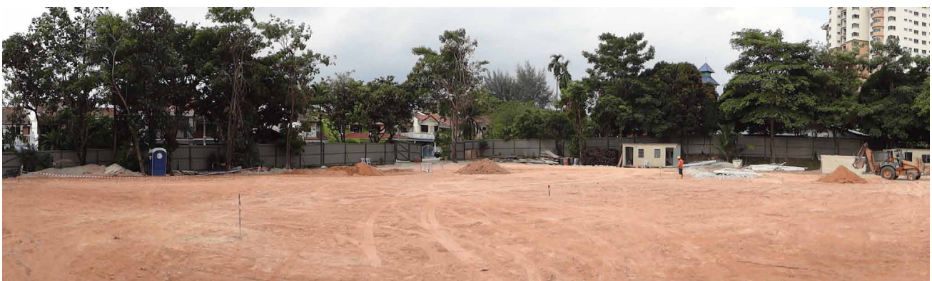
The overview of the overall completed project.
