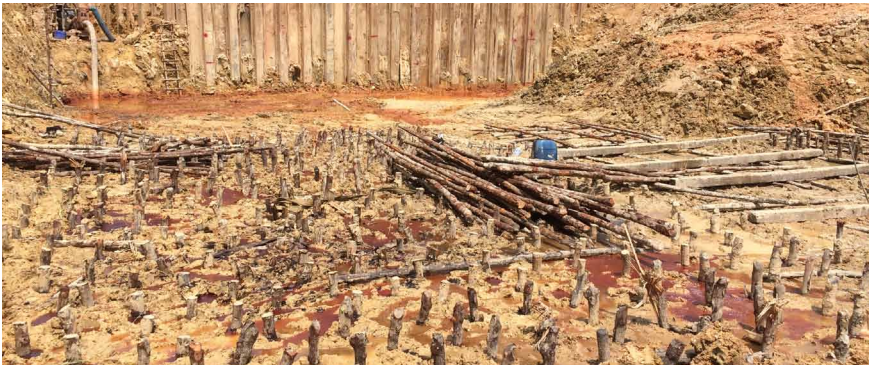
Installation of bakau piles over the soft subgrade.
