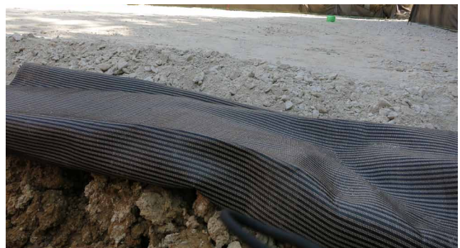
Completed load transferring platform on top of the geotextile.
