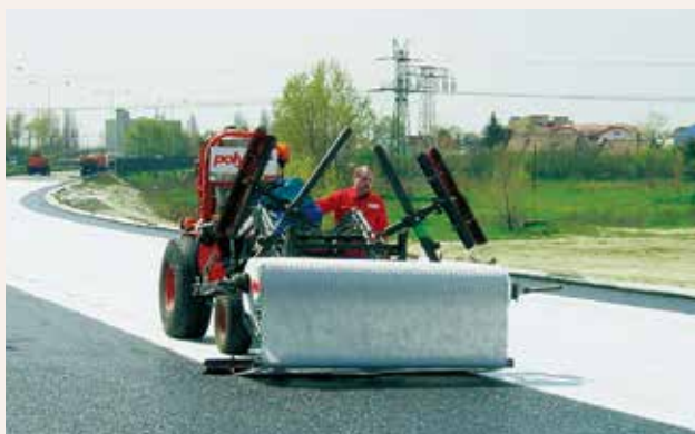
弯道处完美的铺设TenCate Polyfelt® PGM-G
