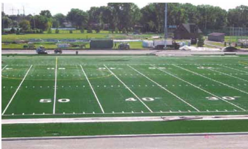
Installation of TenCate Mirafi® FW402.
