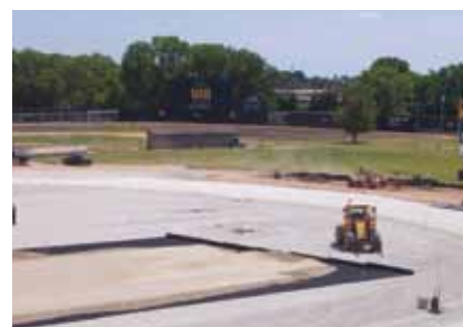
Installation of TenCate Mirafi® FW402.
