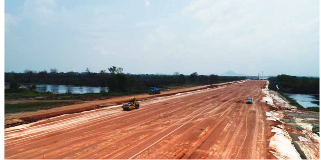
Figure 7. Compaction of embankment fill by heavy machinery
