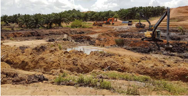
Figure 3a. Soft soil condition on site
