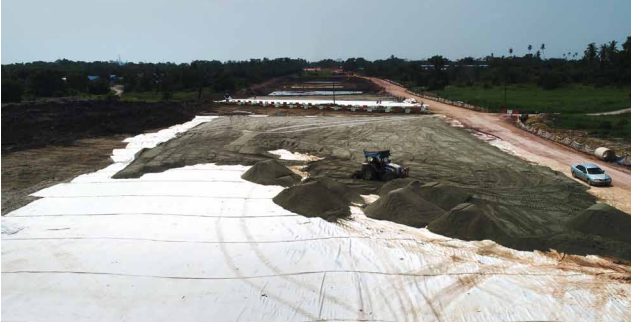
Figure 6. Embankment backfilling on top of TenCate Mirafi® PET high strength geotextile
