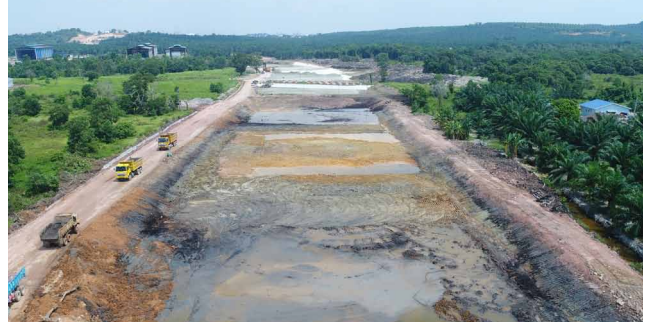
Figure 3b. Soft soil condition on site
