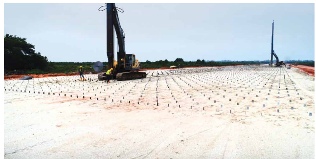
Figure 4. Installation of Prefabrication Vertical Drain (PVD)
