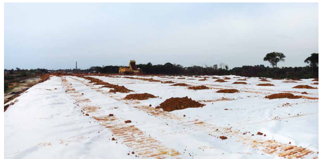
Figure 5. TenCate Mirafi® PET high strength geotextile laid on soft foundation
