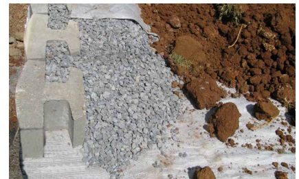
Close up of Polyfelt® PEC and segmental blocks.
