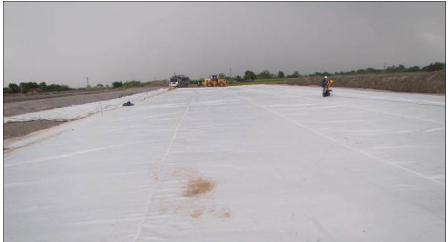
Mirafi® PET 600/50 high strength reinforcement geotextile unrolled over soft foundation
