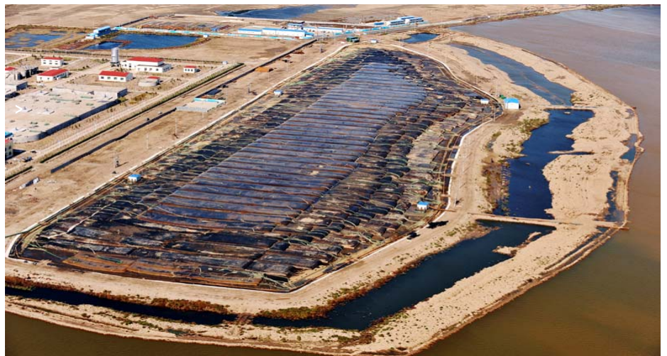
> Figure 2. The Geotube® Dewatering Platform .
