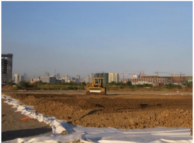
Embankment fill over Mirafi® PET400/50 reinforced geotextile
