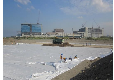
Overview of Mirafi® PET400/50 over soft subgrade foundation
