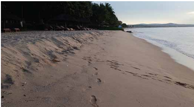
The beach front has been narrowed due to erosion
