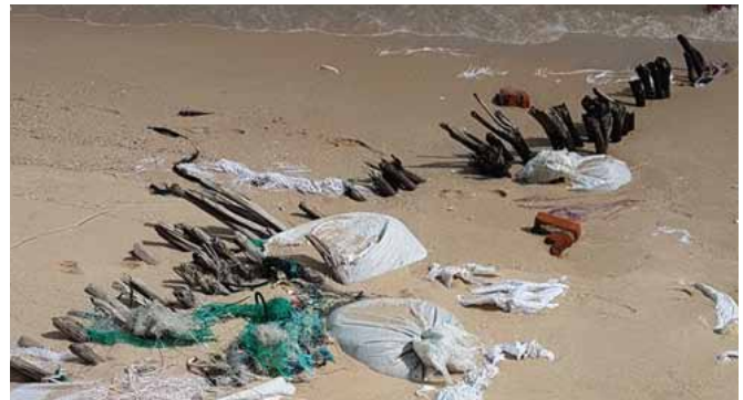
Disintegrated existing conventional plastic sandbag
