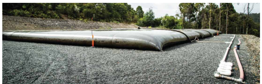
Dewatering of the polishing ponds
