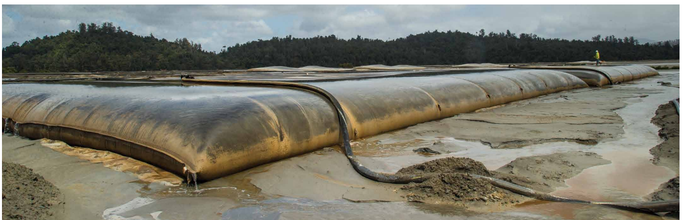
Geotube® units installed over soft tailings
