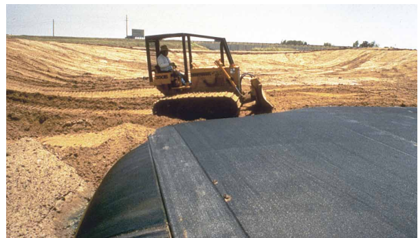
Infilling between parallel fill fingers to complete fill closure
